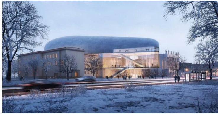
Figure 4.42 : Ostrava Concert Hall, Steven Holl Architects (Url-30).
