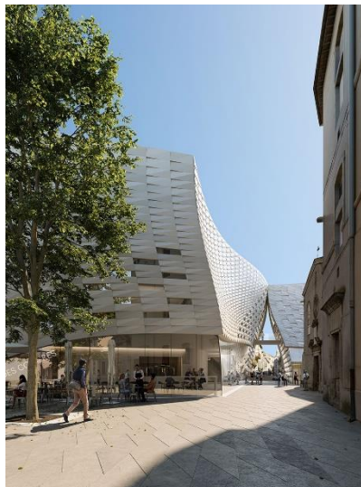
Figure 4.14 : Street and pavement around Palais des Congrès (Url-13).
