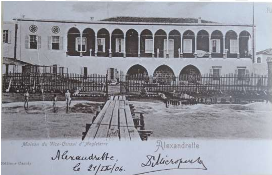
Figure 4.26: Front Facade of the British Consulate on Cayla Boulevard (Şehri- Hatay, p.188)
