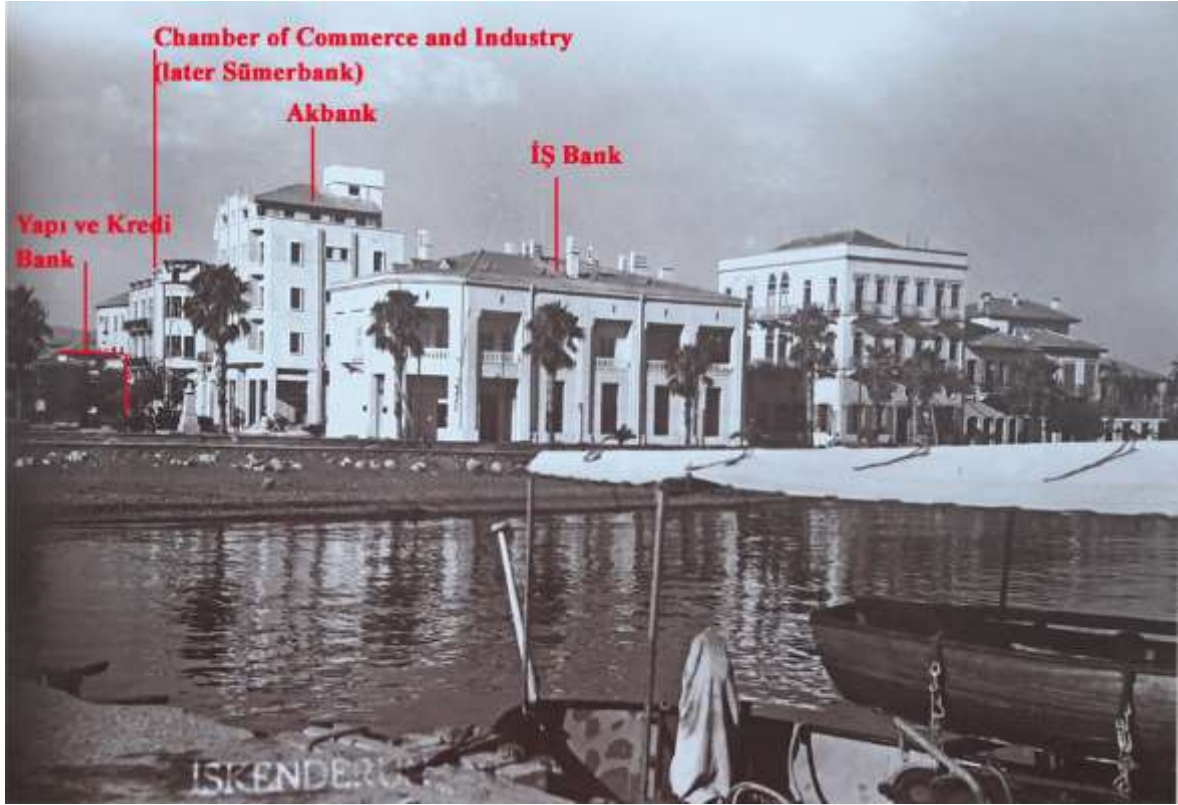
Figure 4.68: The Chamber of Commerce and Industry and the Banks in İskenderun (1952-1958) ( Şehr-i Hatay , p.259)
