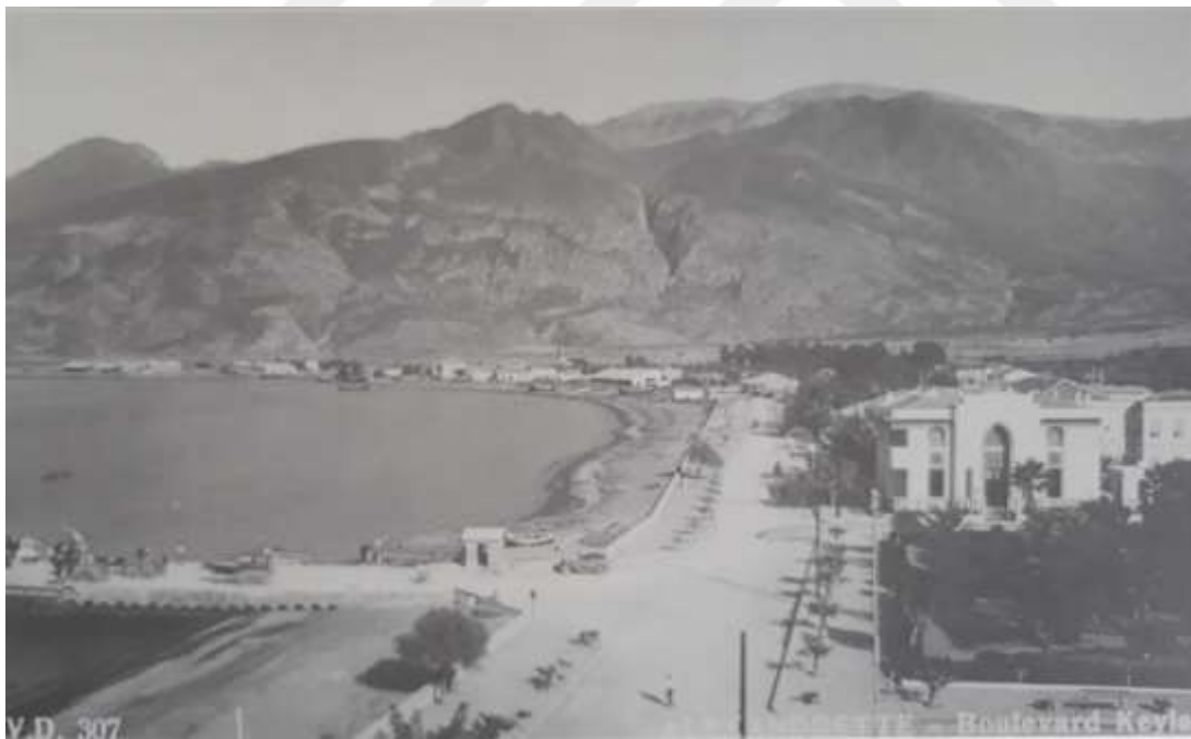
Figure 4.4: The Road Along the Sea Built During the French Mandate Period (Mursaloğlu, n.d., p.54)
