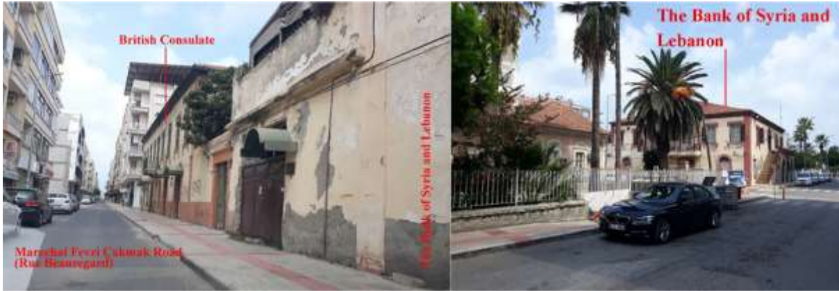
Figure 4.27: The Bank of Syria and Lebanon located on the Rue Beauregard (after 1939 named as Mareşal Fevzi Çakmak Street ) (Photo was taken by the author)
