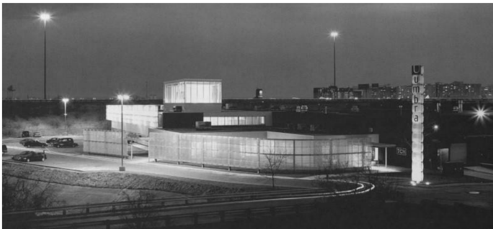
Figure 1.2 : The project reskins an existing warehouse with translucent plastic panels that glow at night (Rappaport, 2003).
