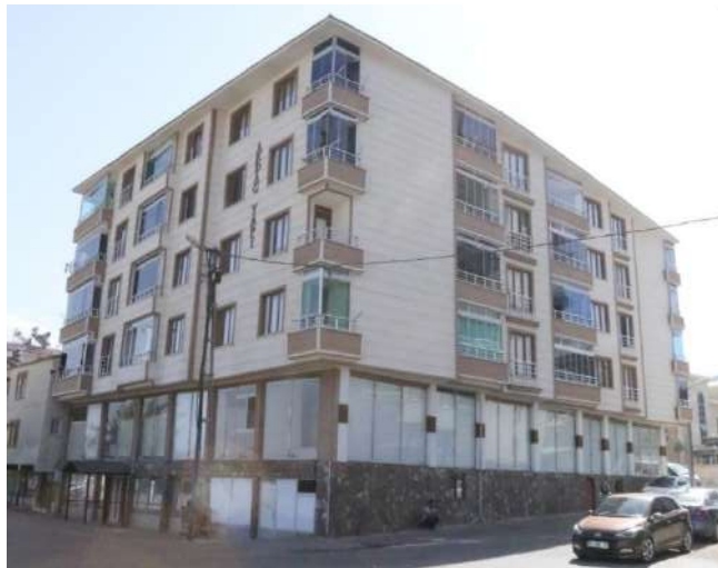
Figure 3.9: Actual image of the project in Genç, Bingöl.
