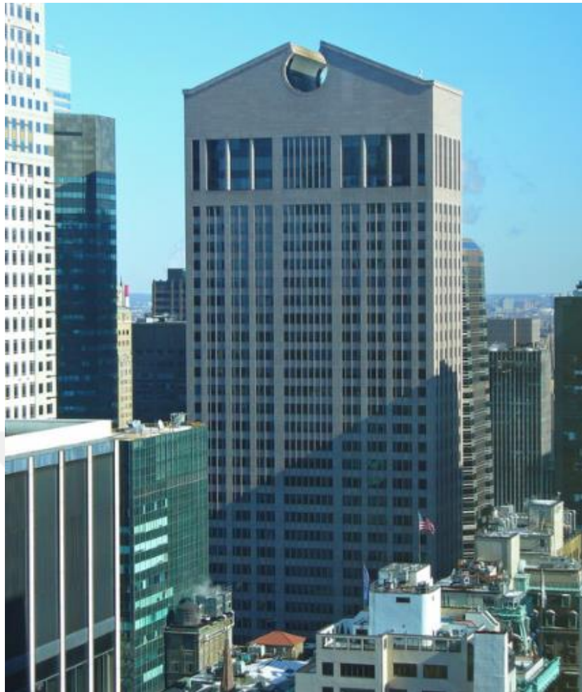
Figure 3. 45 AT&T Corporate Headquarters (Langdon, 2019)
