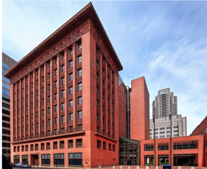
Figure 3. 13 The Wainwright Building (Langholz, 2013)
