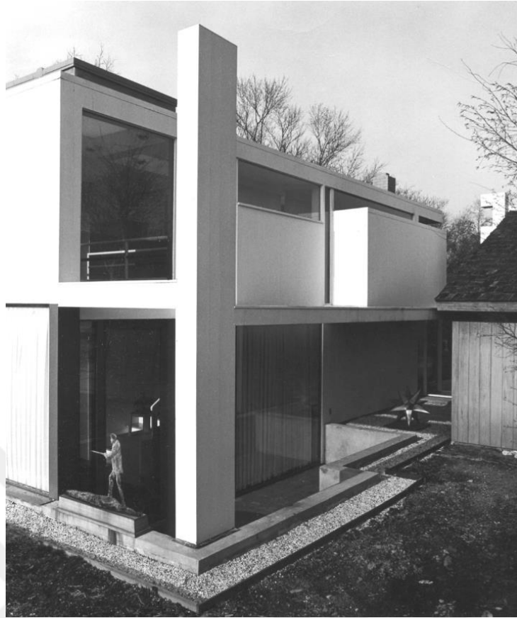
Figure 3. 46 House I (Eisenman, 1968)
