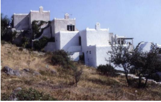
Figure 5.28 : Summer House Complexes Aktur Bodrum. 43
