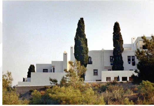
Figure 5.27 : A Photo of Monastery Hotel. 42
