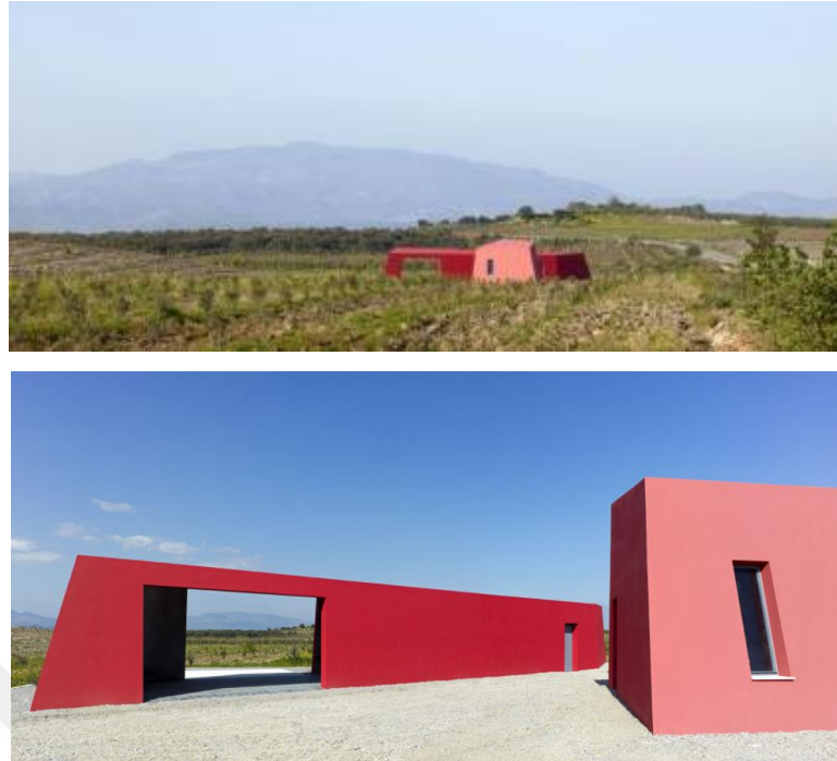
Figure 5.11 : The Warehouse Building in Dikili. 22
