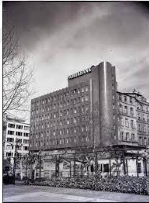
Figure 5.96 : Pamukbank Head Office 117
